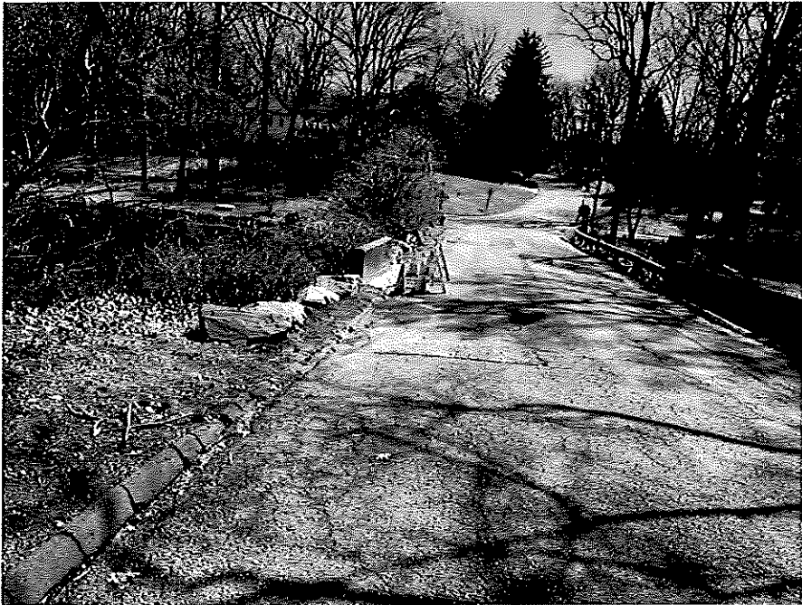
Photograph 5. General View of North Approach, Looking South
