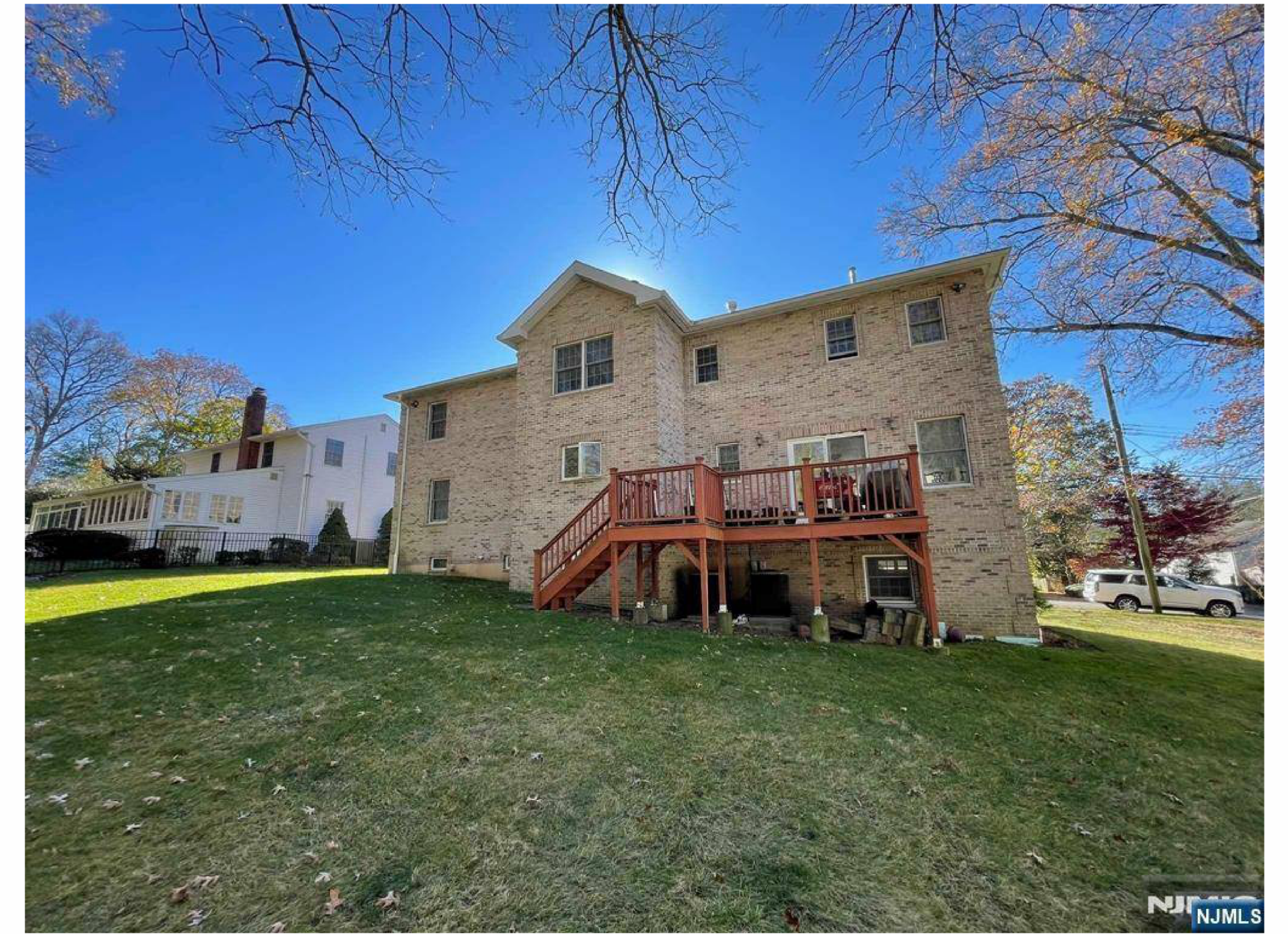
4 EXISTING REAR VIEW
