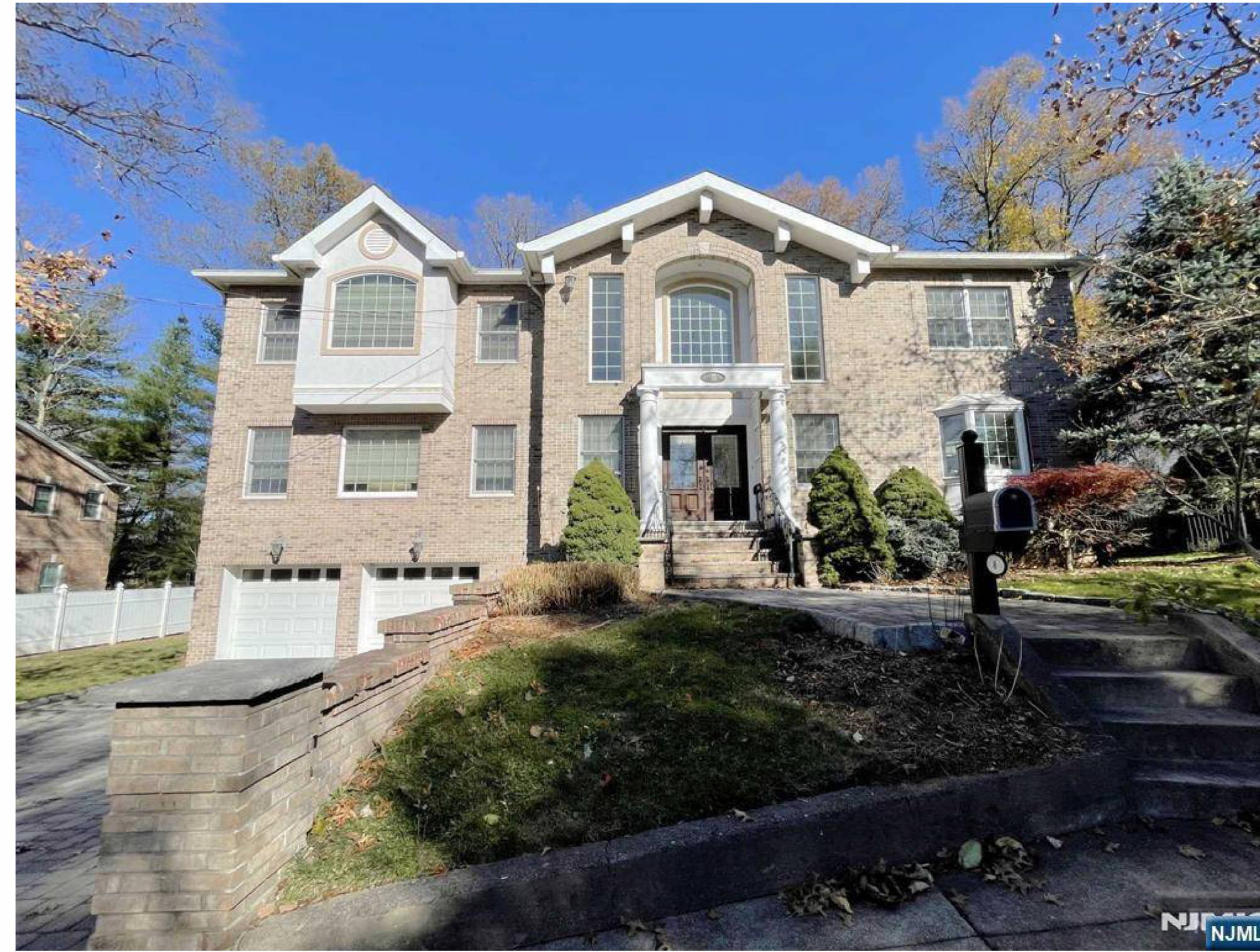
3 EXISTING FRONT VIEW
