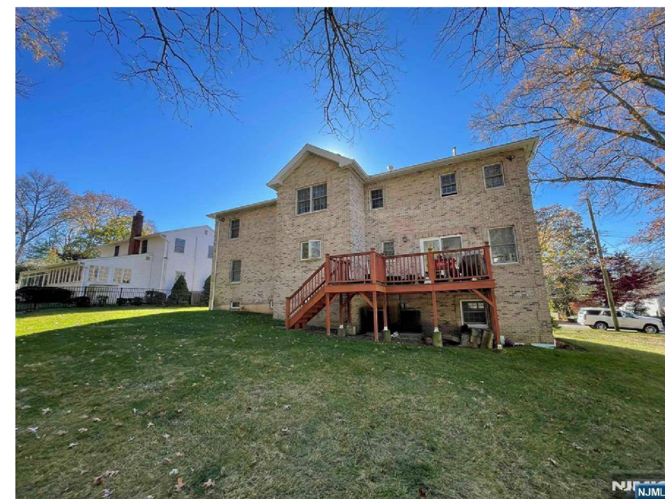
7 EXISTING REAR VIEW 1" = 20'-0"
