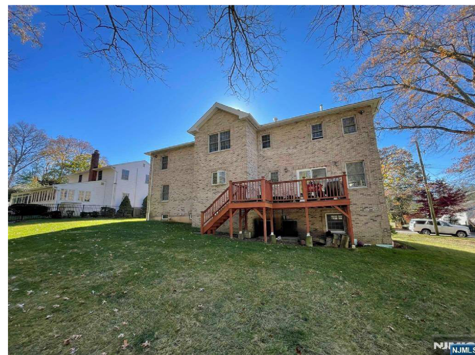
7 EXISTING REAR VIEW 1" = 20'-0"
