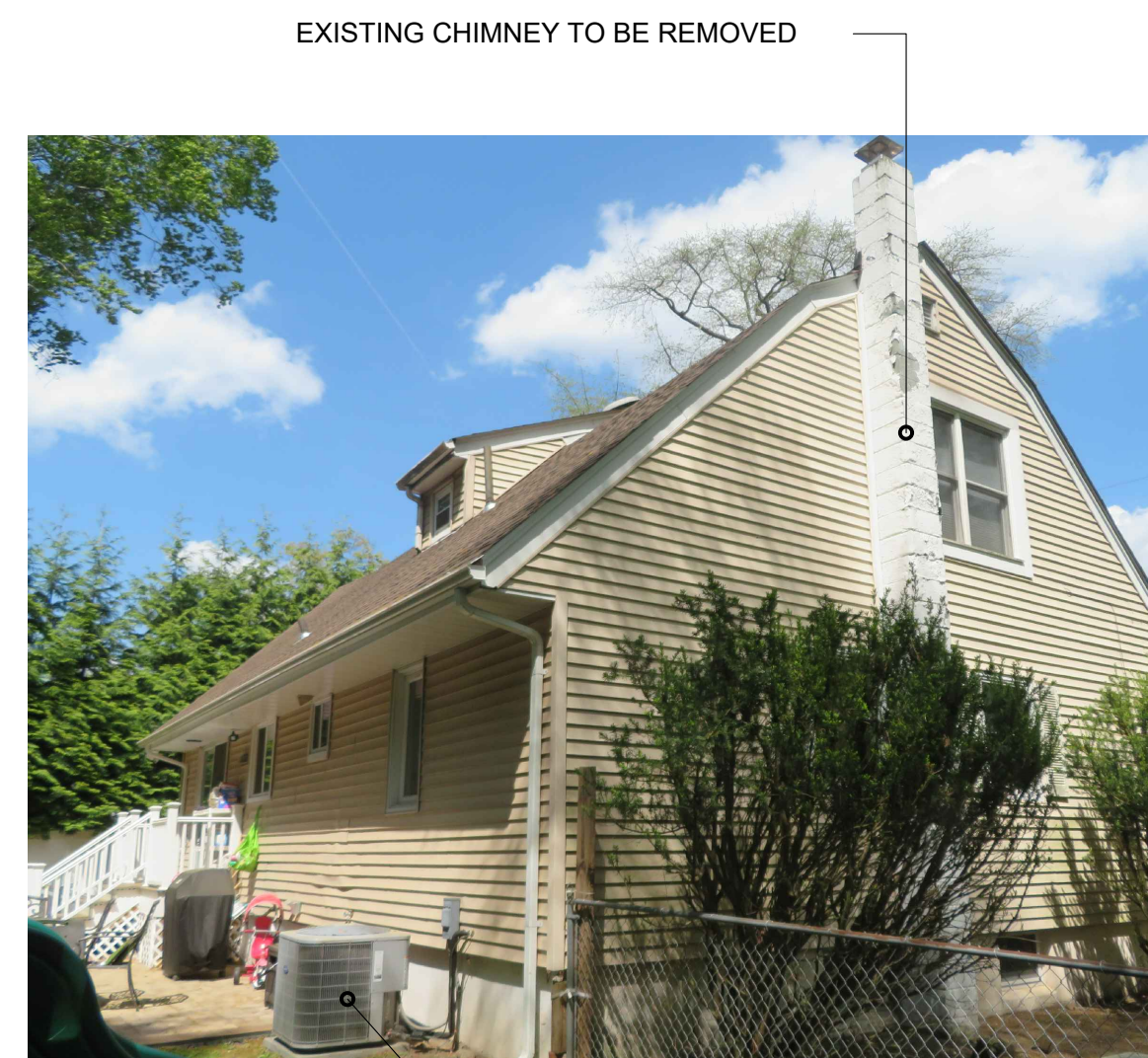
EXISTING PHOTO-3 (FROM WEST, SOUTH)
