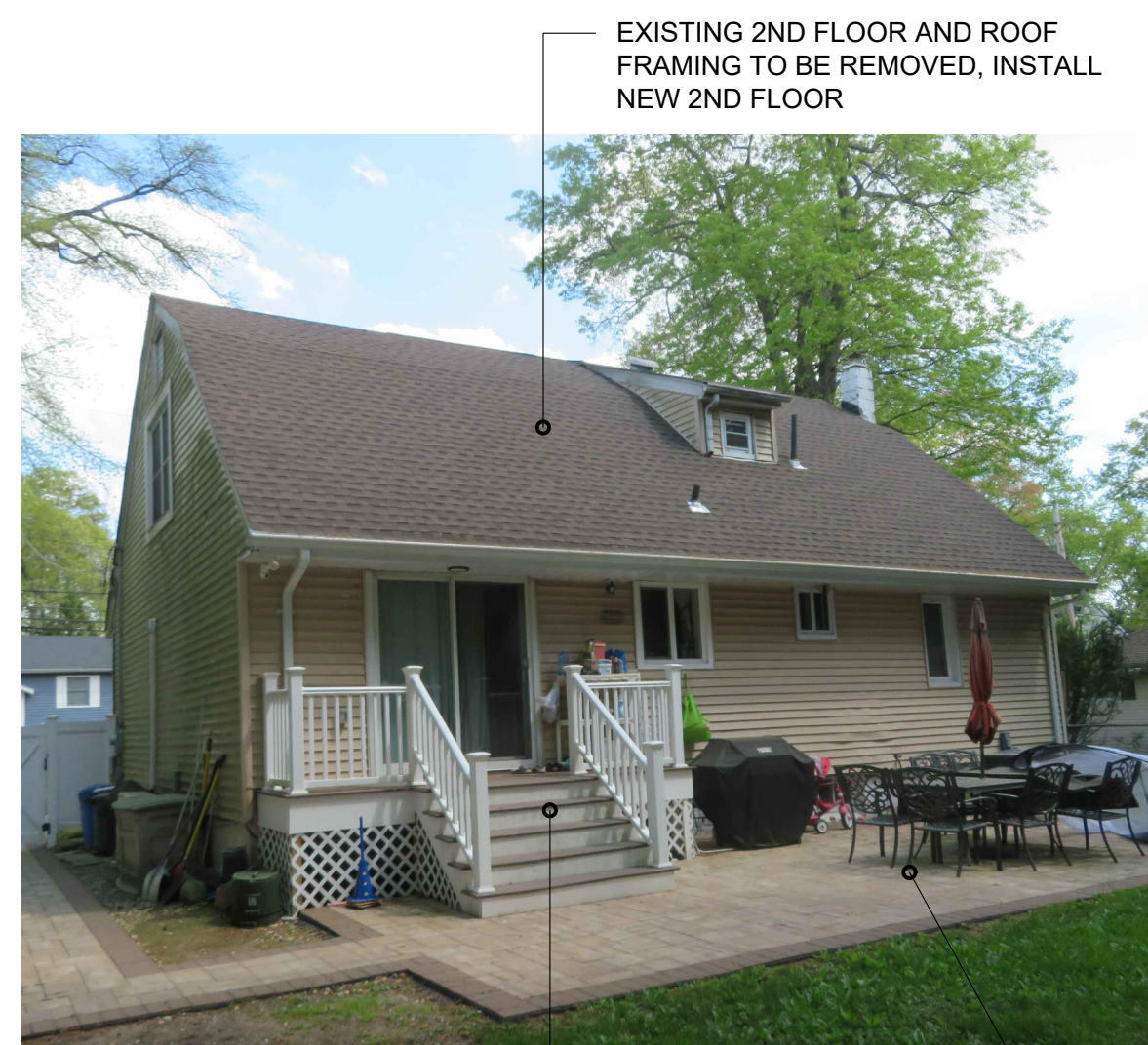
EXISTING PHOTO-2 (FROM WEST, NORTH)
